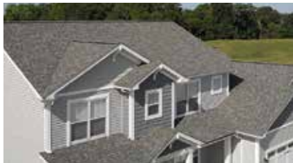
ROOFING AND VENTILATION
